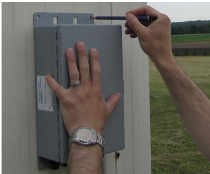
Figure 63: Surface-mounting the enclosure
