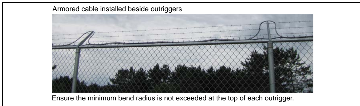
Figure 50: Armored cable installation on barbed wire
