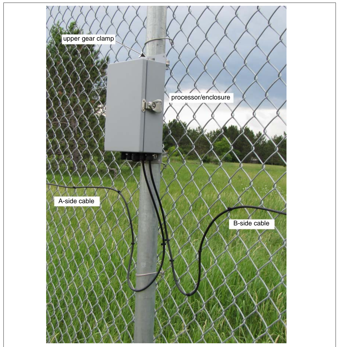
Figure 61: FlexZone single pass dual zone fence-mounted processor
